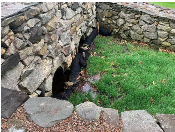
4 Brickyard Circle - 1 (Drainage Course)
