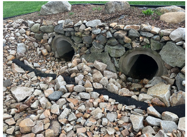
64 Gundalow - 2 (Drainage Course)
