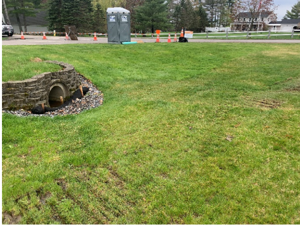
29 Gundalow - 1 (Drainage Area)
