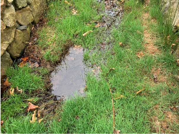
4 Brickyard Circle – 3 (Drainage Course)
