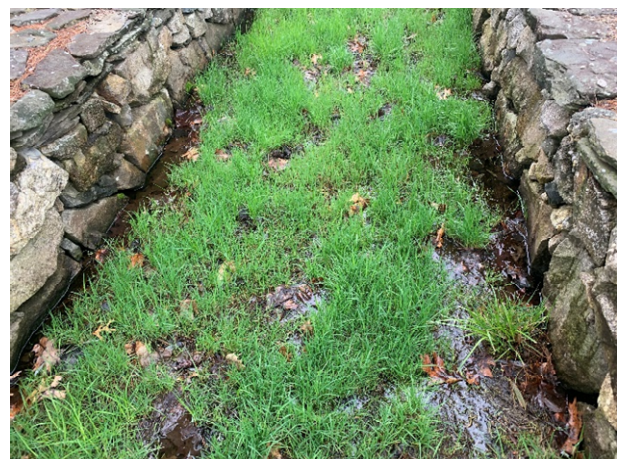
4 Brickyard Circle - 2 (Drainage Course)
