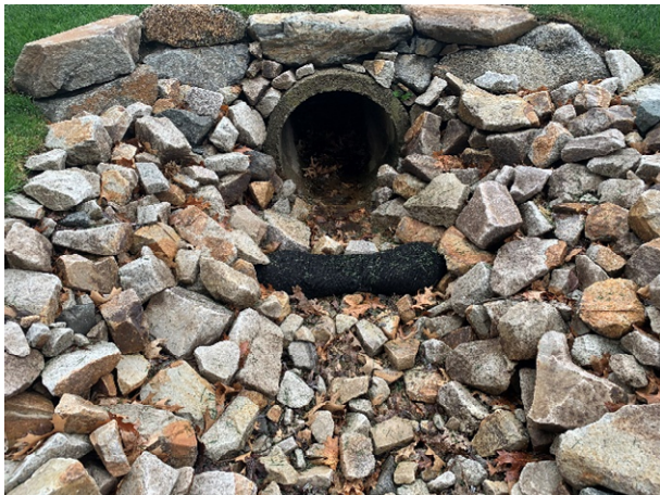
64 Gundalow - 1 (Drainage Course)
